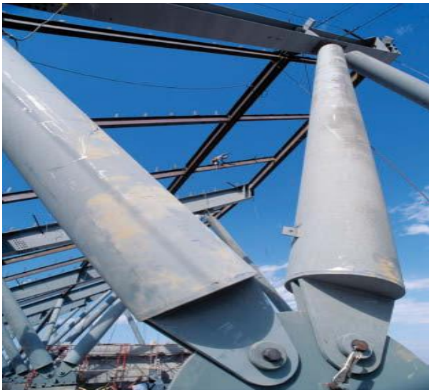
The structural elements in the foreground transmit concentrated forces to the brackets at both ends
