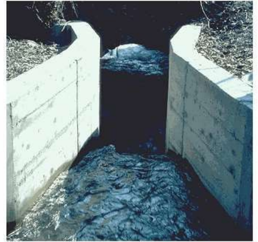
Fig: Triangular weir in minc34 wall and Venturi channel.
