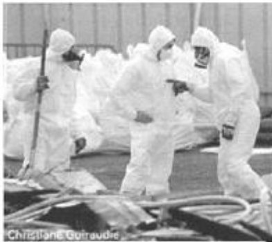
(c) Asbestos decontamination
