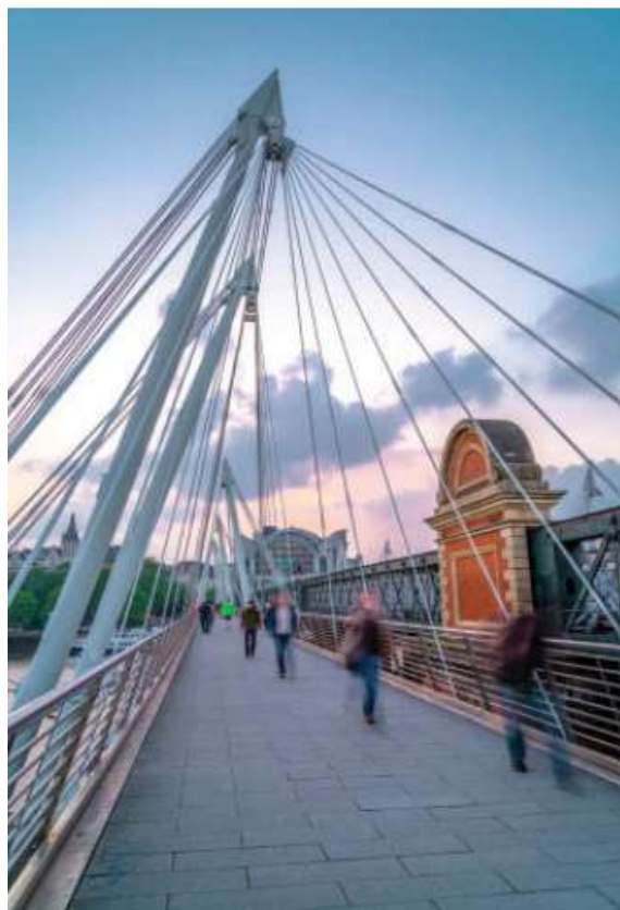
One of the two Golden Jubilee Bridges in London, England, adjacent to the Hungerford Bridge. The cables of this bridge exert a three-dimensional system of concentrated forces on each bridge tower.
