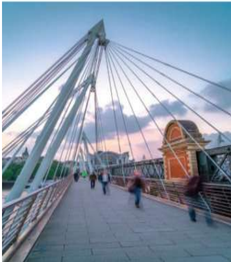
One of the two Golden Jubilee Bridges in London, England, adjacent to the Hungerford Bridge. The cables of this bridge exert a three-dimensional system of concentrated forces on each bridge tower.
