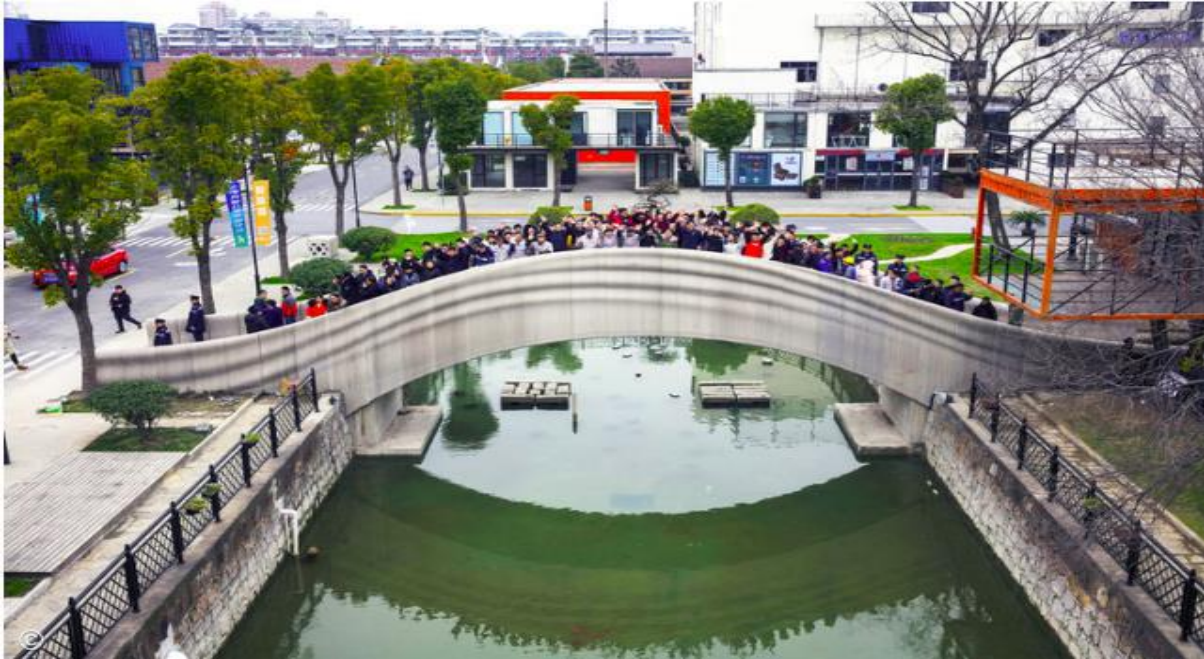
Figure I.8. World's Largest 3D-Printed Concrete Pedestrian Bridge Completed in China.
